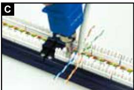
Terminate wires using Linkbasic tool or equivalent.
