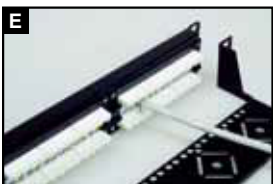
Install the Cat6 rear cable management
